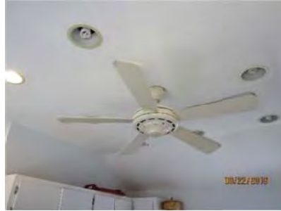
4.8 Fan and fixtures appeared general sound. Exception of some bulbs burnt out. Fan operation was wobbly.
