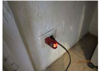
4.42 Closet receptacle outlet appeared generally sound.
