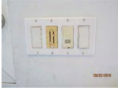
4.7 Switches appeared generally sound
