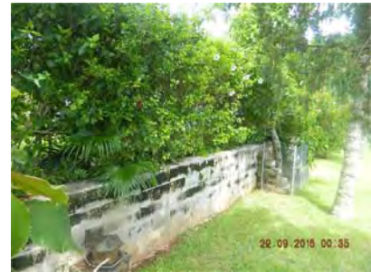
South border retaining wall appears satisfactory
