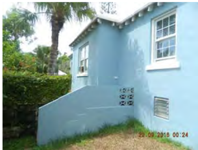
Wall finishes appear satisfactory
