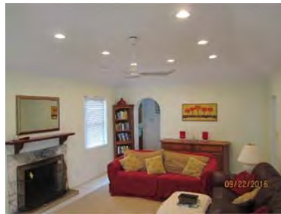
4.20 Living Room fixtures switches and outlets appeared generally sound.
