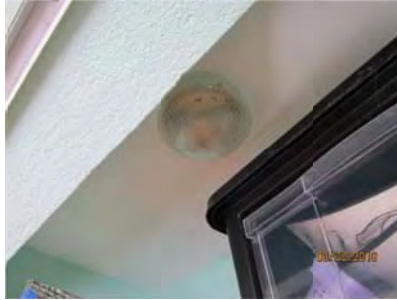
4.35 Closet fixture appeared generally sound.
