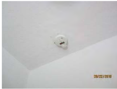
4.56 Smoke detector tested ok appeared generally sound.
