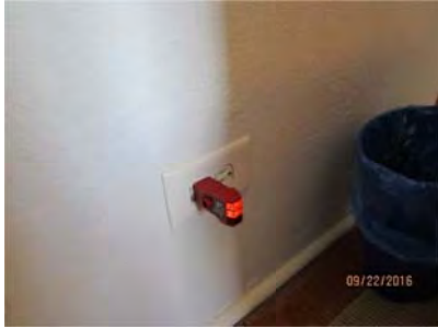
4.52 Receptacles outlet appeared generally sound.
