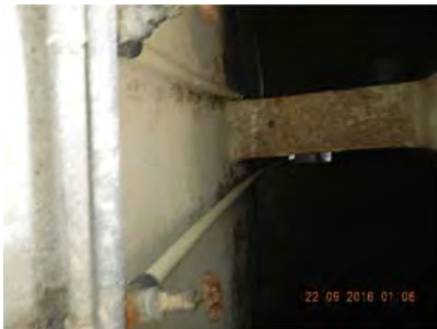
Tank view looking down at divide walls.
