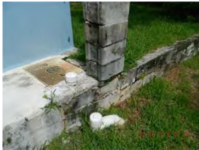
Cesspit clean out and vent. Drop off step may be a safety hazard.
