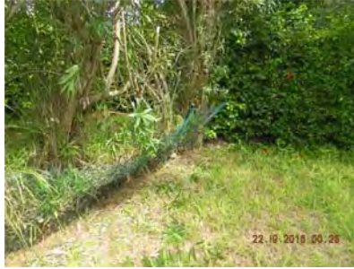
Chain-link fencing/posts need repair.
