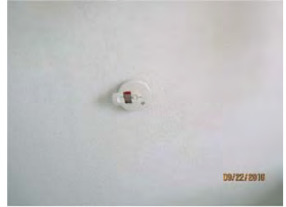
4.36 Smoke detector appeared generally sound.
