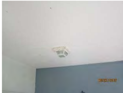
6.2 Fixture south porch appeared generally sound.
