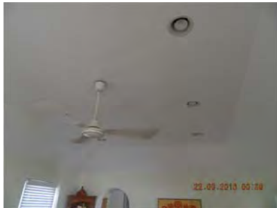
Living room ceiling appears satisfactory
