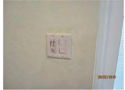
1.27 Switches appeared generally sound.
