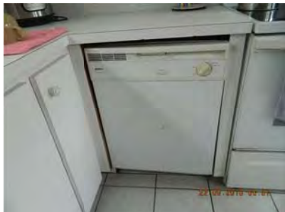
Dishwasher needs repositioning and securing to cabinets/countertop
