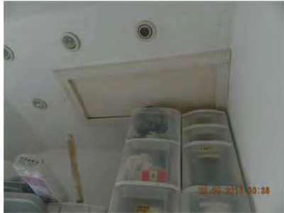
Laundry scuttle hatch not accessed.
