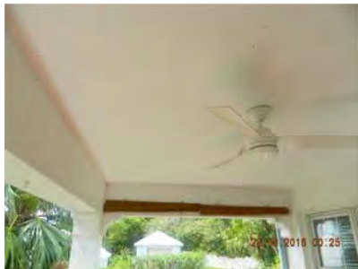
Porch ceiling is satisfactory
