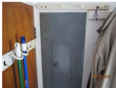
3.3 A 30-CCT 120/240V Sub panel located in the laundry. Appears generally sound.
