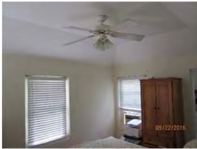
4.37 Master Bedroom fixtures, switches and outlets, smoke detector appeared generally sound.
