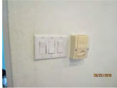
4.26 Switches appeared generally sound.
