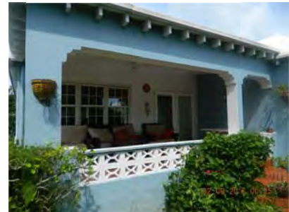
Porch beams and columns appear satisfactory
