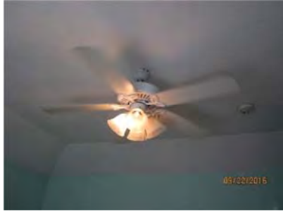
4.34 Ceiling fan and light appeared generally sound.
