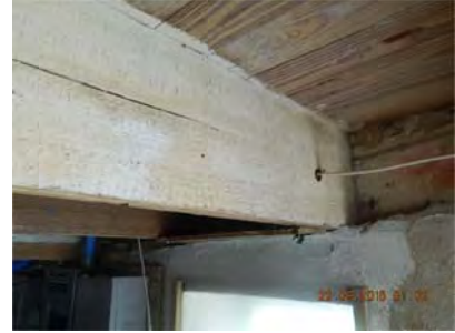
Floor joists appear satisfactory
