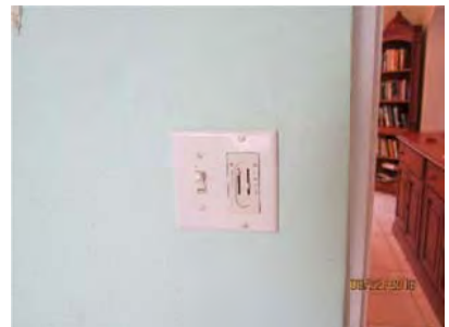
4.33 Switches appeared generally sound.
