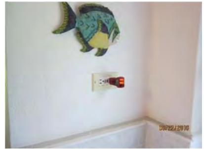
4.48 GFCI tested outlet ok. Appeared generally sound.
