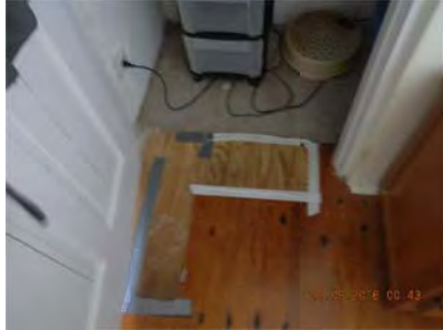
Floor repair needs finishing
