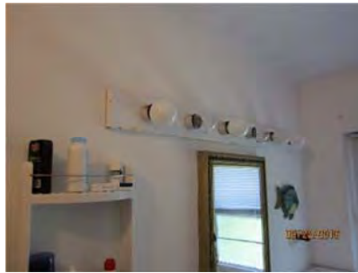
4.47 Hallway Bathroom fixtures switches and outlets appeared generally sound.
