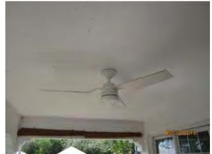
6.3 Fan south porch appeared general sound.
