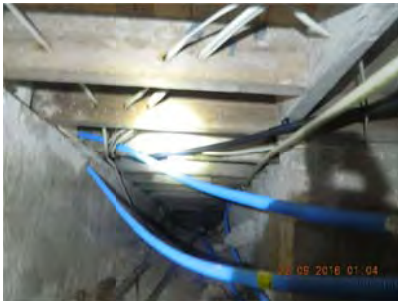
Floor joists viewed in cellar appear satisfactory
