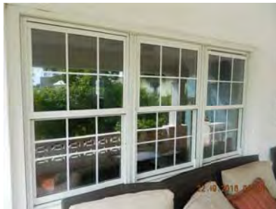
Aluminium windows are functional but need adjustment
