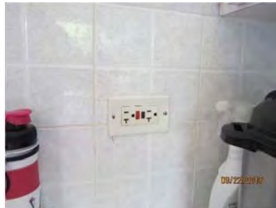
4.5 GFCI west wall tested ok
